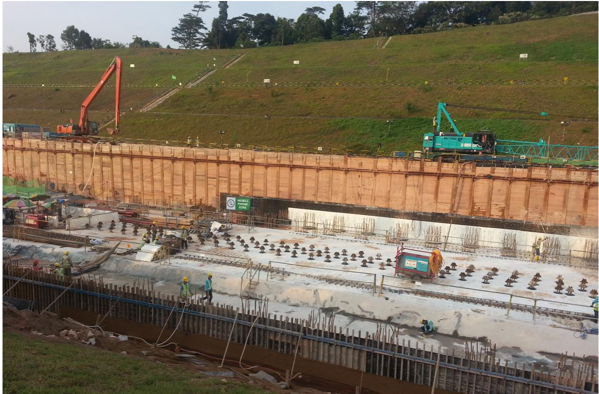
Figure 9. Soldier Pile and Timber Lagging Wall with Open Cut Excavation
