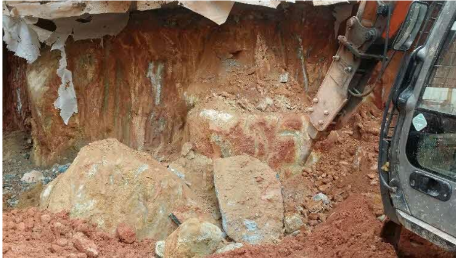
Figure 13. Boulders broken by hydraulic breakers
