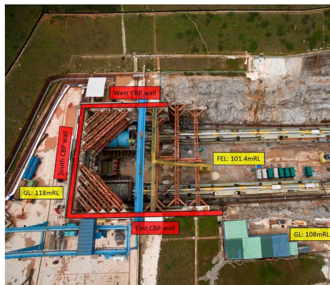
Figure 10. Plan View of the Launch Shaft
